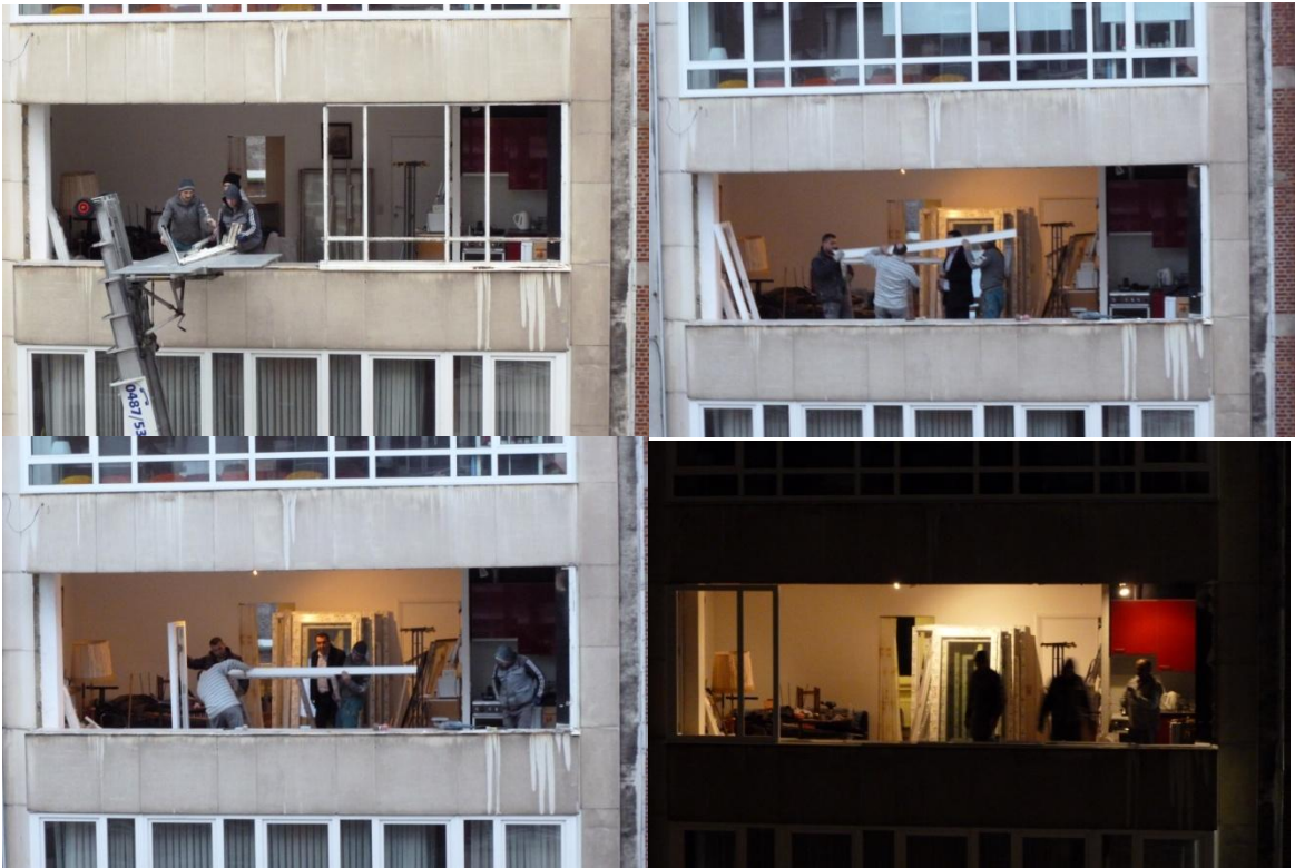
Figure 4: Window assembly on the first day.
