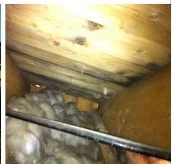
Old insulation, mold in roof due to limited ventilation
