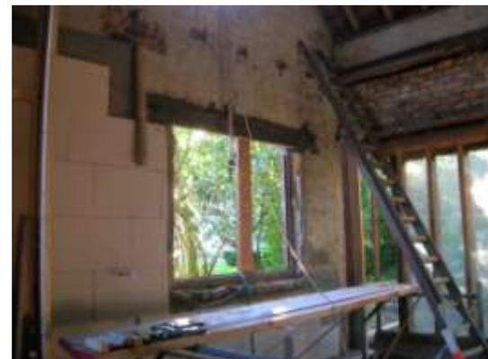
*Interior insulation of the walls. As protected building it was impossible to exterior insulation. This means more thermal bridges to treat.*
