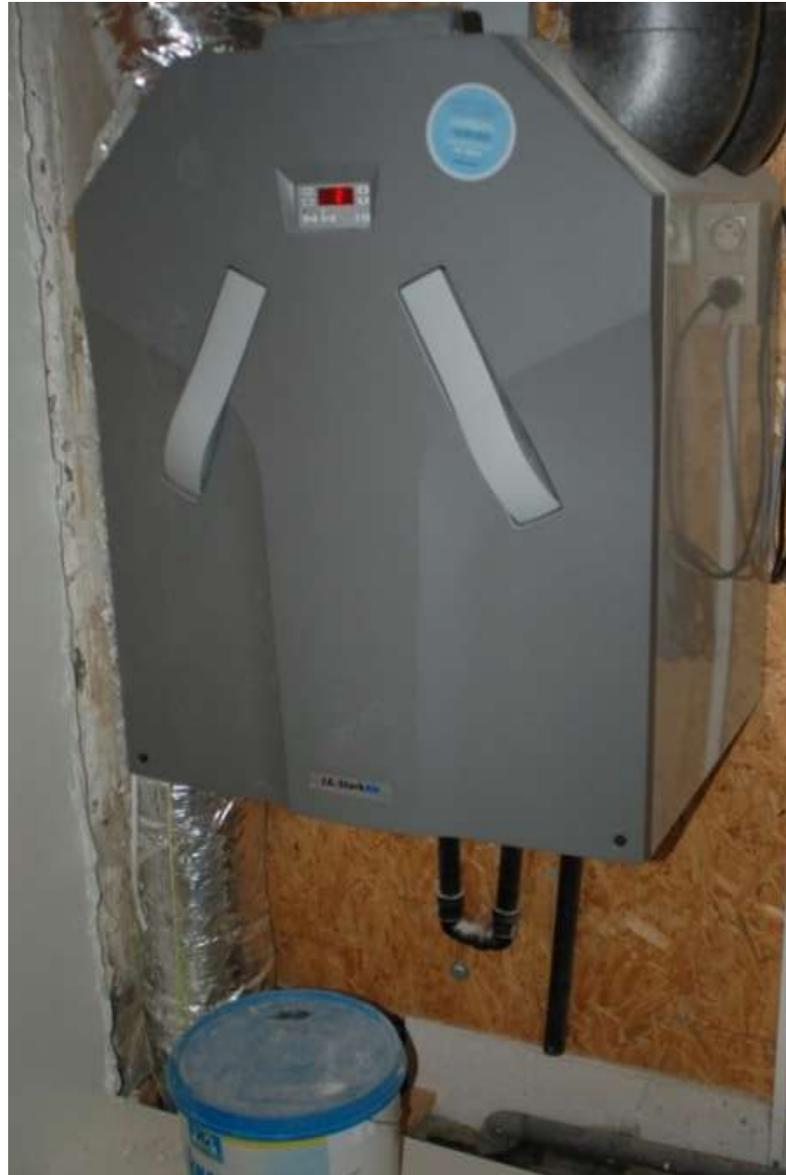
Ventilation system D – with heat recovery
