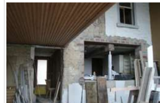
Image during the renovation
