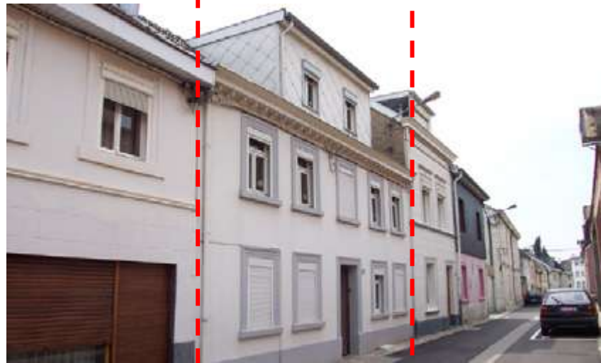
Façade before renovation
