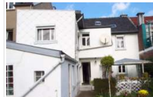
Back façade before renovation
