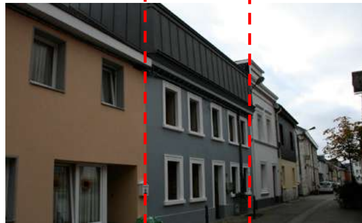
Façade after renovation
