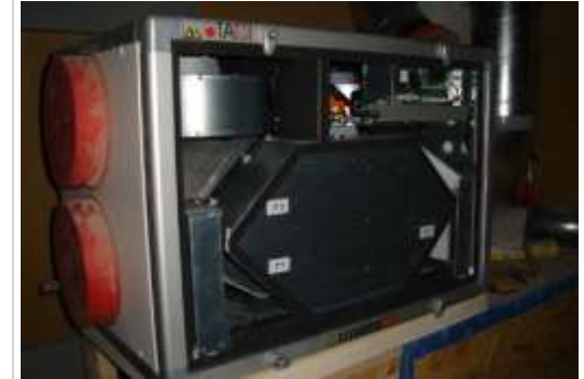
Ventilation system "D" with heat recovery (R=78%)
