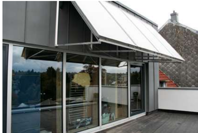
Solar collector as solar shading
