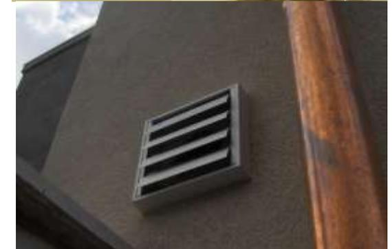
Exhaust fan with humidity dedection in the bathroom and exhaust ventilation grille in the rear façade.
